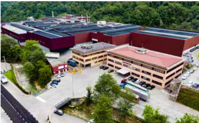
Via Malpaga 82, 25070 Casto (BS) Italy Loc. Ferriera 5, 25070 Casto (BS) Italy A.I.A. n. 1389 del 19/06/2020
